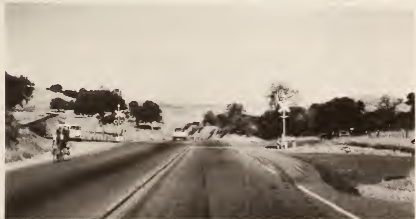
Figure 57 Driver View - 200 Feet (61m) (Amador Central Crossing)
